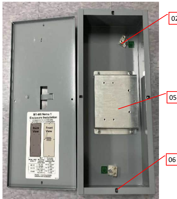
Photo 2 - Internal view of enclosure
